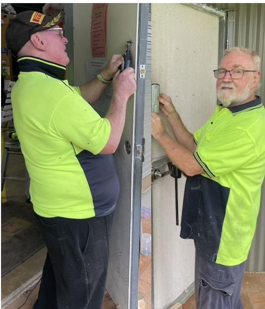
Code Lock Installation: From Left, Warwick Mitchell & Mal Darwent
