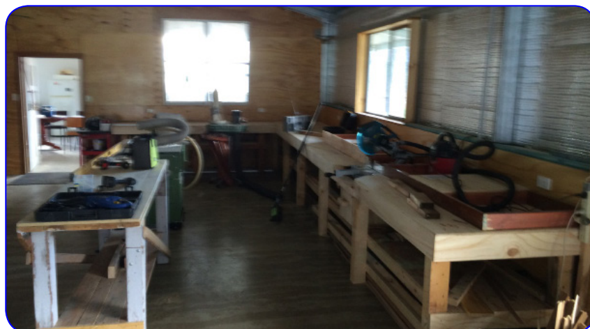
Workshop outfitting well on the way – July 2015
