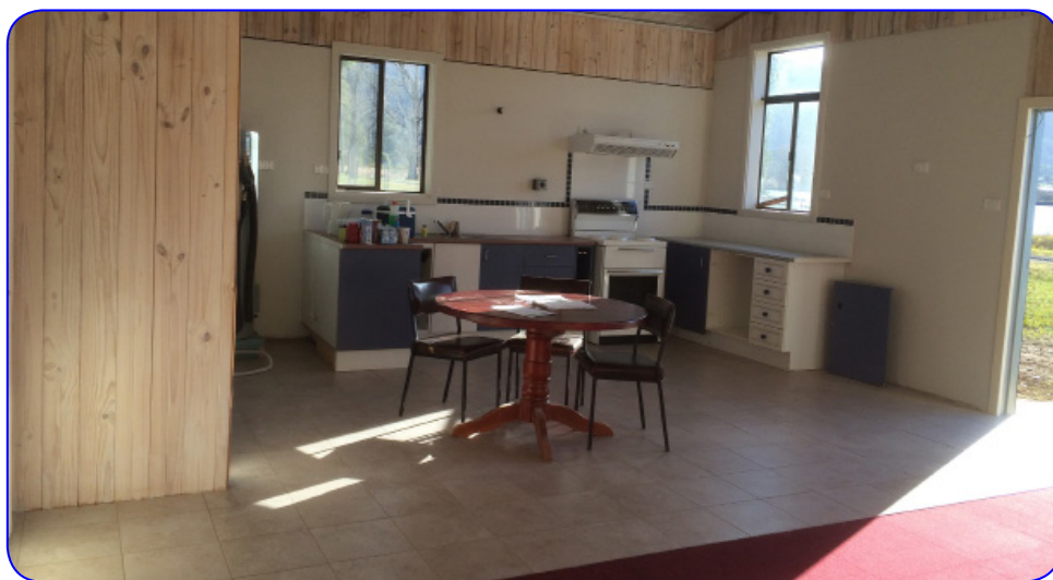
Kitchen & Recreation Area nearing completion – July 2015
