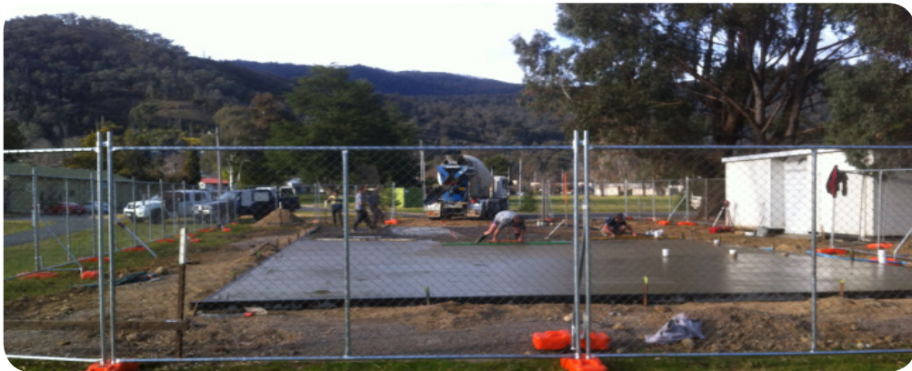
It's happening — foundations
