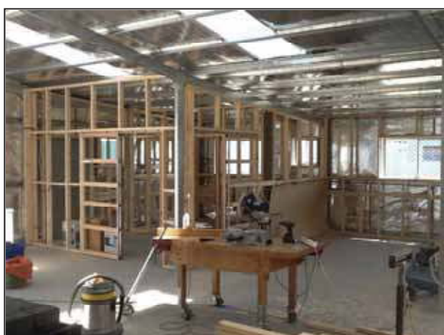
Fitting out of the toilet
